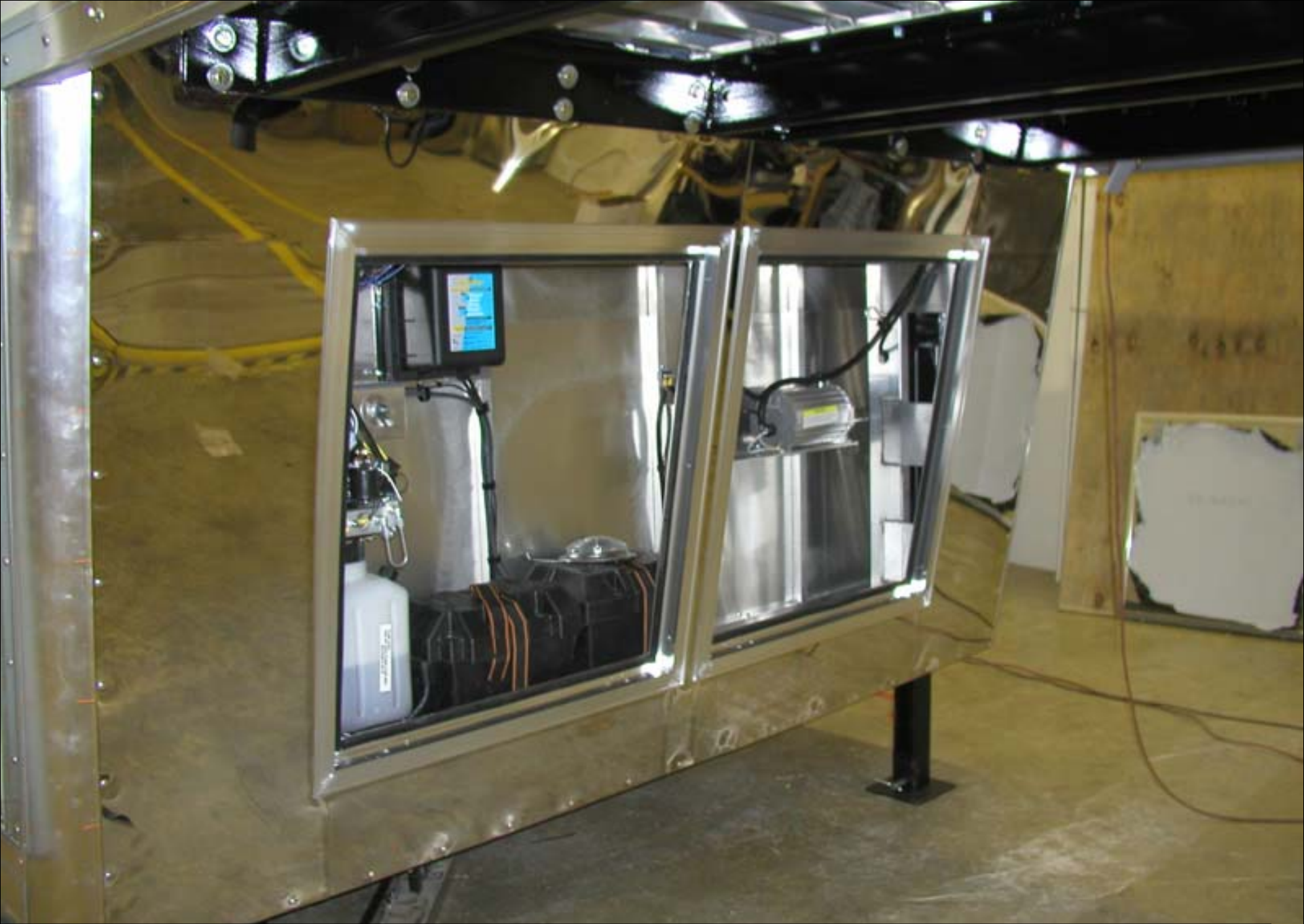
FRONT EXTERIOR COMPARTMENT UNDER UPPER DECK AREA
